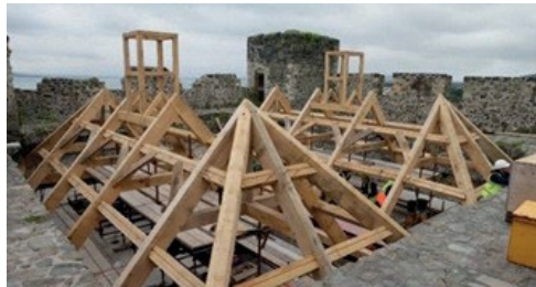
Carrickfergus Castle, Great Tower- roof replacement
